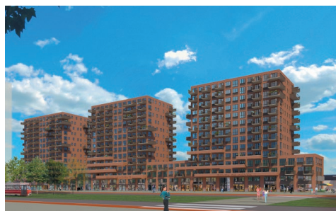
Webo manufactured the cladding panels for the three residential towers in Delft. The cladding panels were lifted by a crane and screwed to place from inside.
